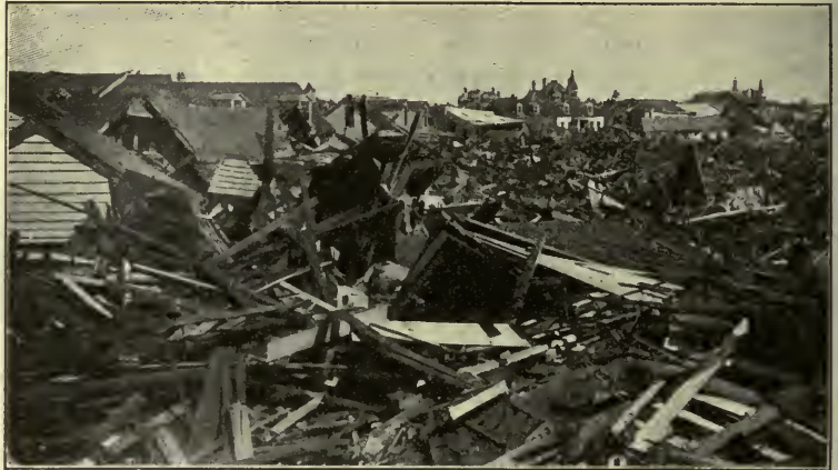
FIG. 412. — A scene in Galveston, Texas, showing the vast destruction done by a hurricane in 1900, when many of the houses were torn to pieces during the storm.
